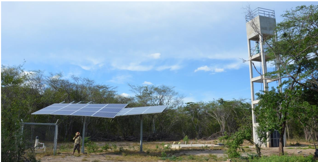
Figure 42: Well with photovoltaic system, treatment system and water tower
